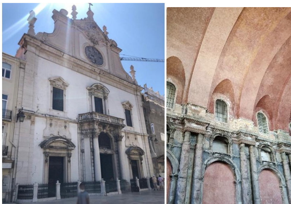
Figure 3: St. Dominic Church (M1 & A2), from left to right: a) rebuilt exterior of the church; b) marks of the fire inside the church
